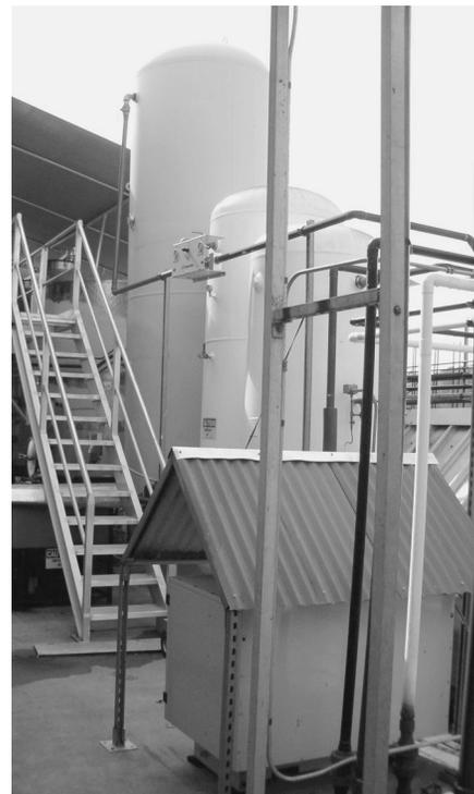
**Kunde Winery installed a new 15hp air compressor to replace a 50hp compressor and added a second, larger 2,560-gallon air holding tank to the existing 1,670-gallon tank in 2004. The increased air-holding capacity allows a smaller air compressor to run less often while maintaining a constant pressure.**
